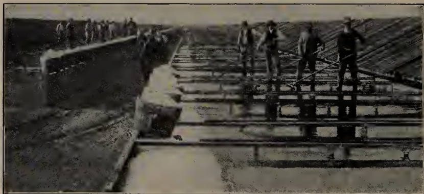
FIG. 161. The evaporation of salt brine in the open air
